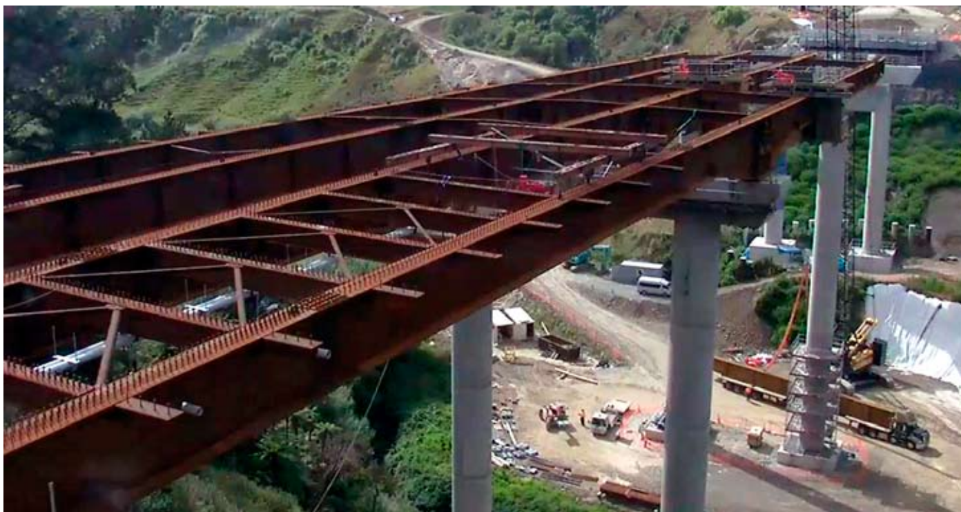
The Cambridge Bypass composite bridge.
