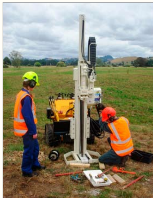
LAL's Environmental Group installs a shallow groundwater monitoring well using drill mast and skid steer.
