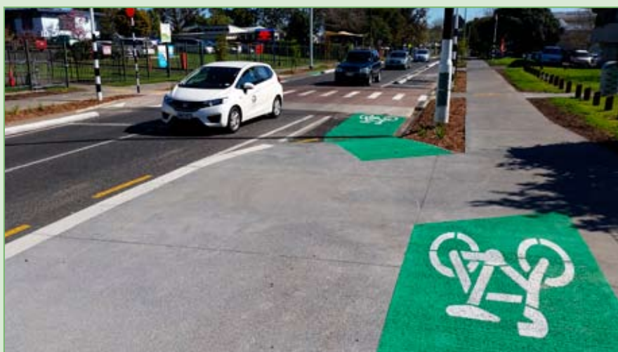
An example of the Future Streets treatments showing the widened footpaths, raised crossing, separated cycle lanes and approach to a prototype bus stop. The treatments include a two-kilometre 'community circuit'.
